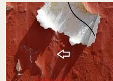
Adhesion Failure
