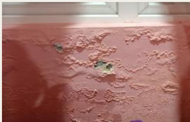
Efflorescence Failure
