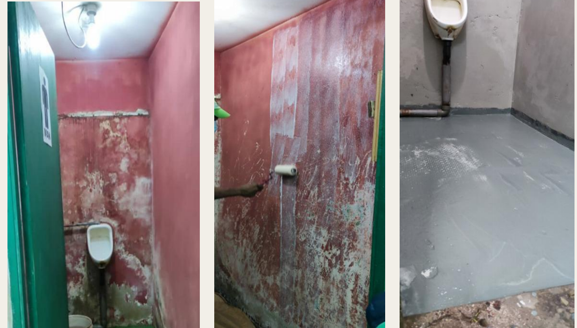
Cementitious Waterproofing Applied at Toilet Area
