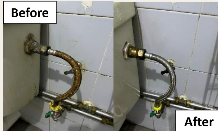
Washroom Stain Surface Cleaning
