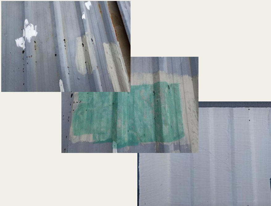
Waterproofing on the metal roof repairing
