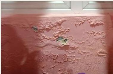
Efflorescence Failure
